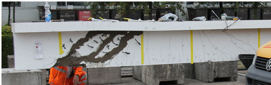
Fig. 14. Beam 1 after failure tests. Injected shear cracks. The repaired beam was designated as Beam 4.
