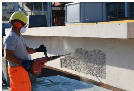
Fig. 2. Concrete hammering on one of the test beams.
