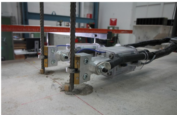
Fig. 10. Detail of the cooper clamps for the connection of the electric power supply (resistive heating) with the U-shaped memory-steel stirrups on Beam 2.
