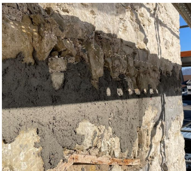
Sections in the middle are filled with mortar
