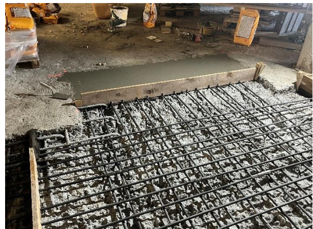
Grouting with SikaGrout®-314 N
