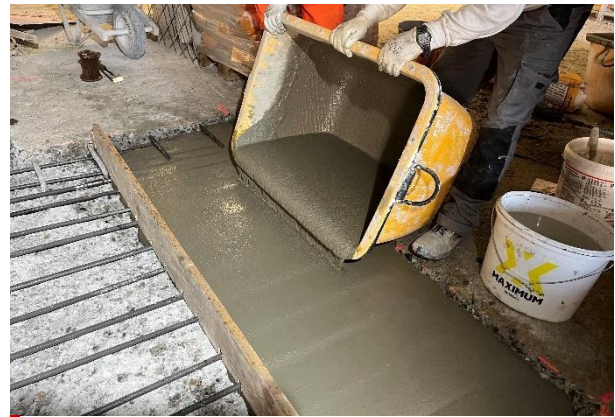
Grouting the anchoring areas
