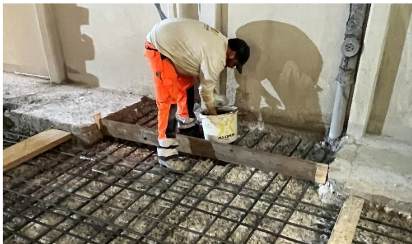
Preparation of formwork
