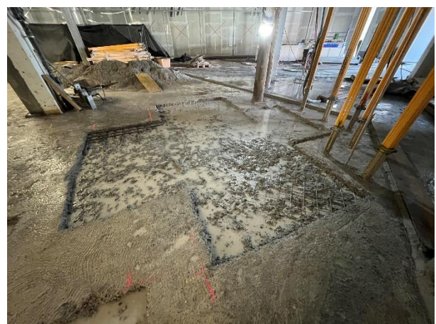
Reinforcement areas, waste disposal
