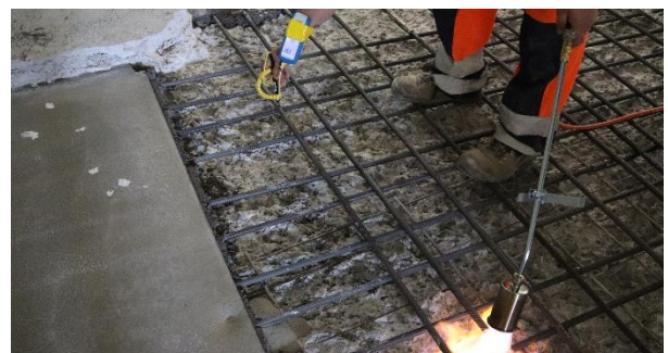
Activation of re-bar with gas and temperature control
