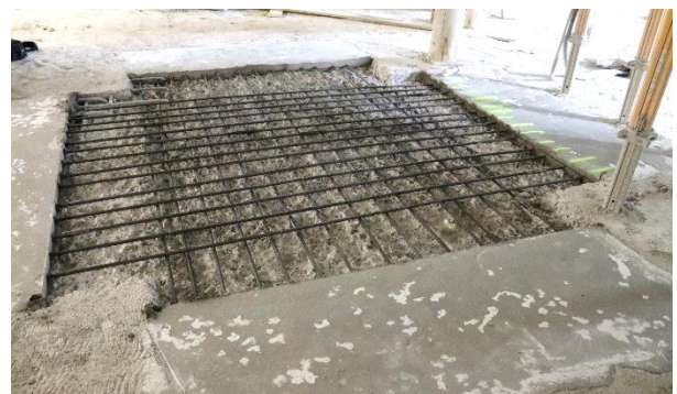
Hardened anchoring areas
