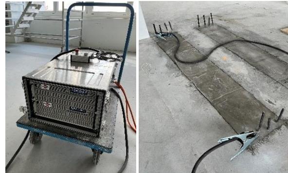
Electric heating device for resistive heating (only handled by re-fer technician)
